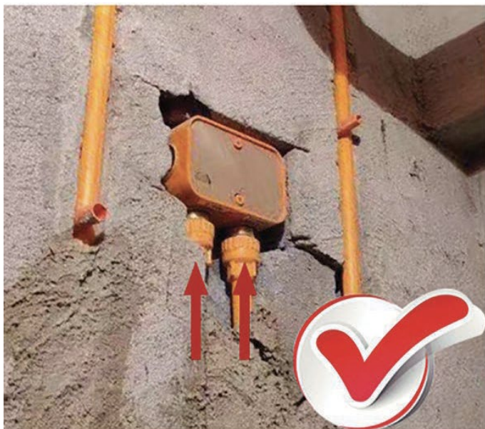
The installation of concealed plastic box in right way
