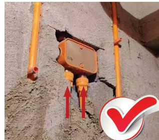
The installation of concealed plastic box in right way
