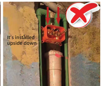
It's installed upside down The installation of concealed plastic box in wrong way
