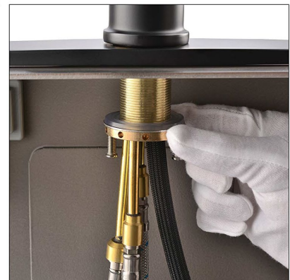
3 Notice: plastic washer is on the top, then the metal collar, the metal nut at the end .
