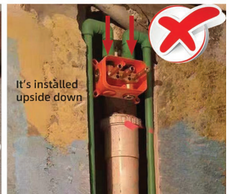
It's installed upside down The installation of concealed plastic box in wrong way
